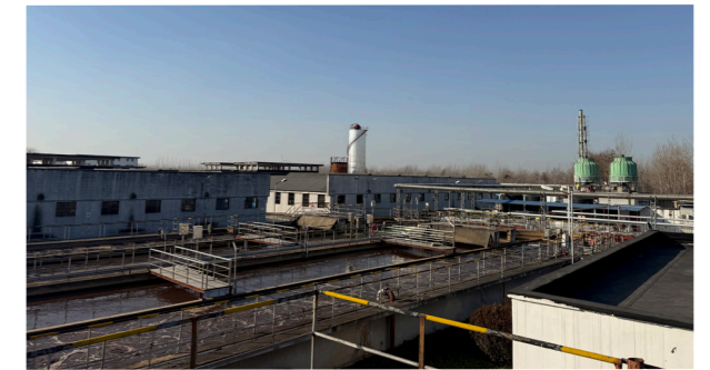
Wastewater Treatment Station
