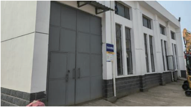
Wastewater Treatment Station
