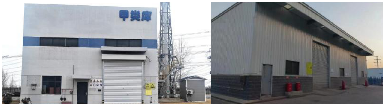
XCMG Machinery Hazardous Waste Warehouse
