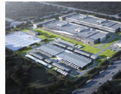
The Company completed delivery of intelligent systems for two Alibaba data centers in the first half of the year. Meanwhile, it delivered complete integrated solutions for China United Yanggao, Yuxian, and Qianqi data center parks, offering efficient and stable O&M solutions for ByteDance.
