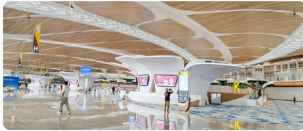
Guangzhou, Construction of Building Equipment and Energy Management Platform for T3 Terminal of Baiyun International Airport and Charging Pile System in Flight Area
