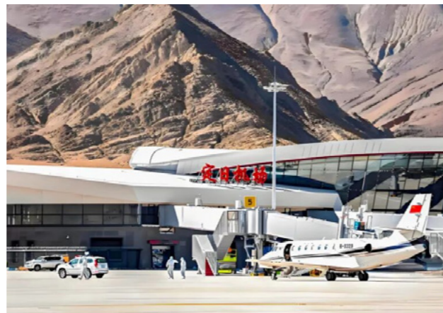
Shigatse Tingri Airport PDMS & EMS Construction
