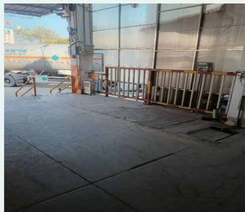
After completion of rectification
