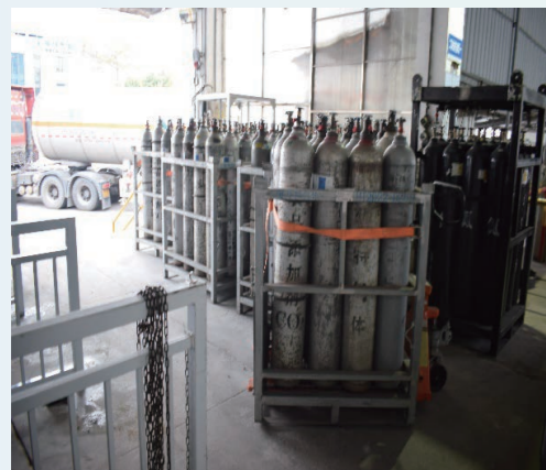
Identification of safety hazards (a large number of cylinder frames were placed on the evacuation passage in the bulk gas workshop)
