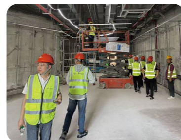
Project Site Inspection
