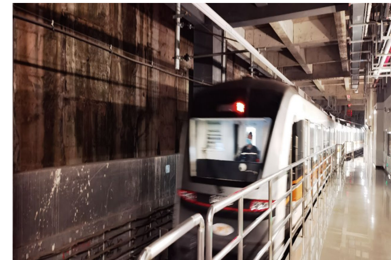
Signaling System for Chongqing Rail Transit Line 4
