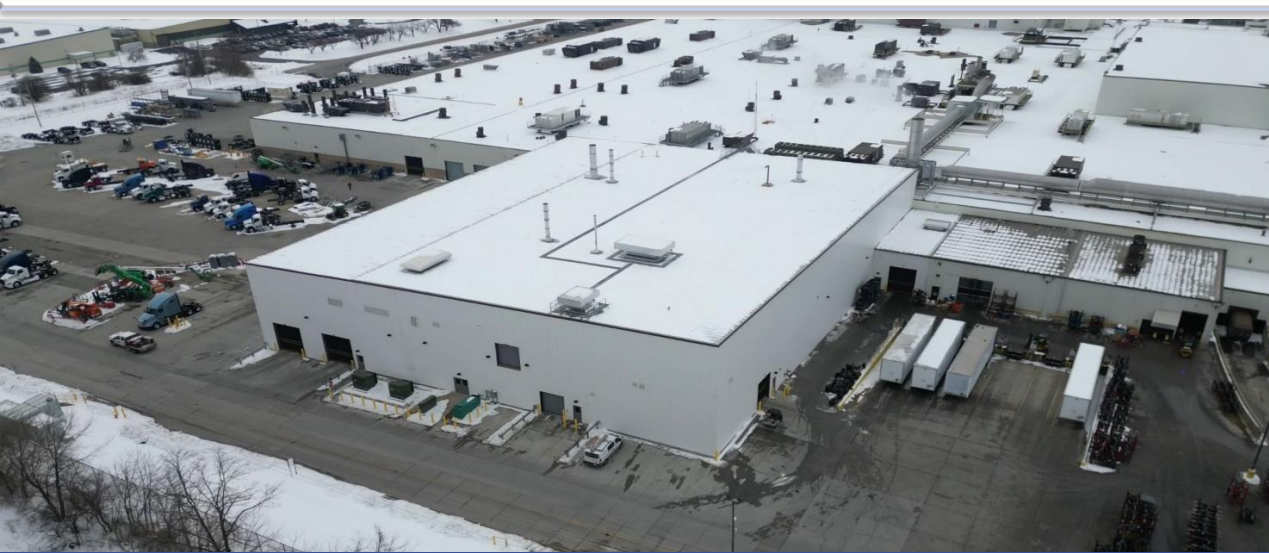
Chassis Paint Booth, Chillicothe, Ohio
