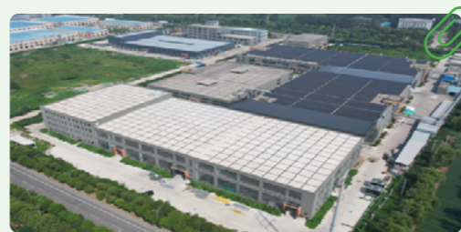
Rooftop Distributed Photovoltaic Project of Jiangsu Advanced Materials
