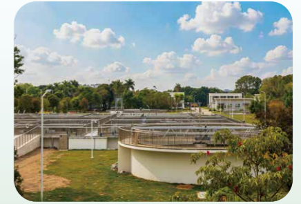
Baiyun Airport Sewage Treatment Plant
