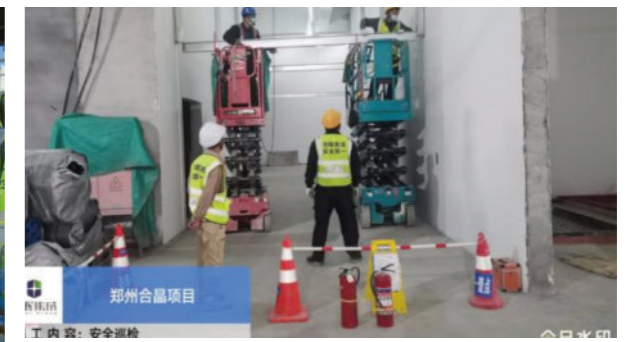
▲ Equipping Protective Equipment
