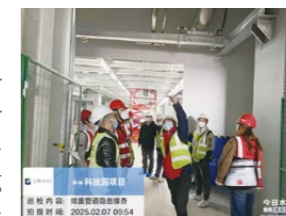
▲ Investigation of Hazards in Waste Discharge Pipes
