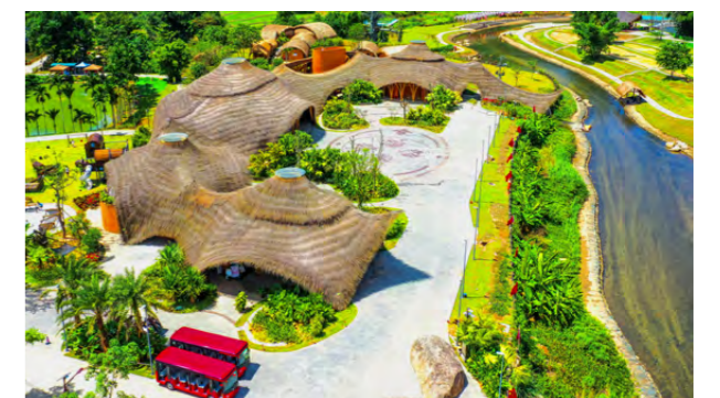
中交路建承建的毛纳村旅游提升项目 Tourism Upgrade Project of Maona Village Undertaken by CCCC Road & Bridge International Co., Ltd.
