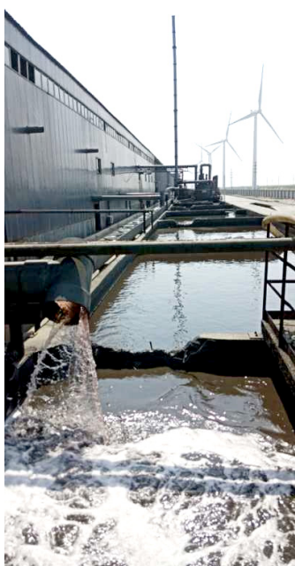
Circulating pool 循環水池
