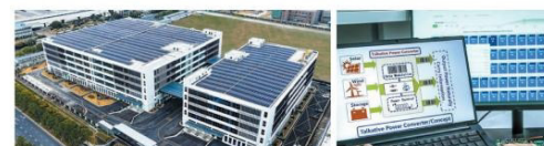
Zhejiang University spinoff company, Hoymiles, is powered with roof-top distributed solar (left). Talkative power converter (TPC) technology, developed at Zhejiang University, is used to control the solar system (right). TPC promises to improve efficiency, reliability and safety of solar power.
