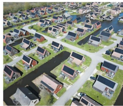
Photovoltaic panels on houses in the Netherlands. Zhejiang University spinoff company, Hoymiles, provides microinverters—components that switch solar DC to AC to power homes or for the grid—in the US and Europe.
