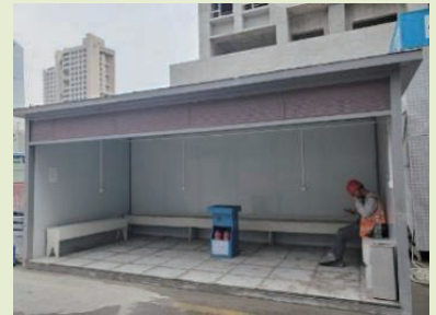
Workers' Rest Shelter 工人休息棚
