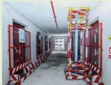
Elevator Shaft Protection Measures 電梯井防護措施
