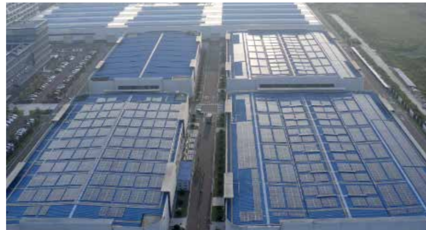
Photovoltaic equipment at Jiangsu base
