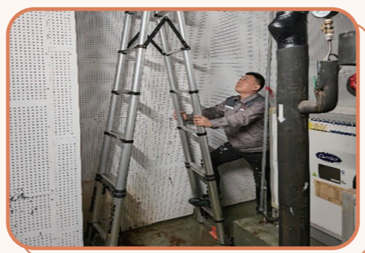
风机房空调检修
