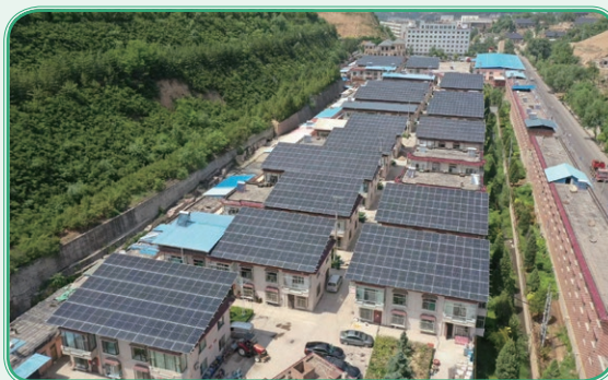
Picture: Jinjiazhuang Coal Mine Roof Distributed Photovoltaic Power Generation Project
