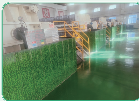
Picture: Coal Tailings Filter Press System Upgrade
