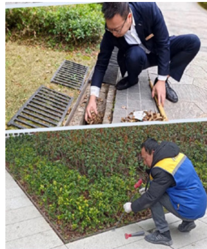
Drainage Ditch Garbage Cleaning 排水溝垃圾清理
