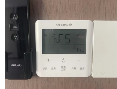
A/C Temperature Not Lower Than 26° C
