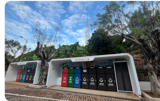
Marubi Industrial Park Waste Sorting Station
