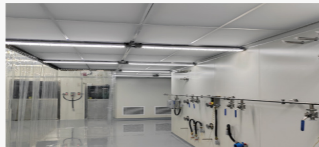
Class 100 Electronic Chemical Reagent Filling Workshop Project
