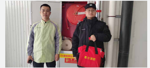
Targeted Fire Alarm Response Test
