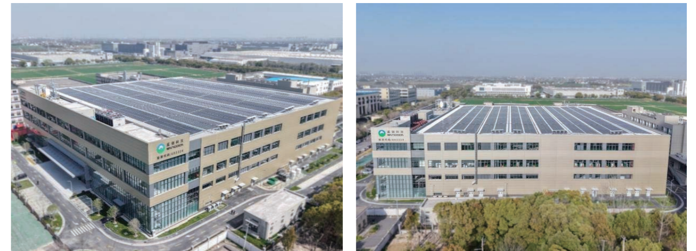
Photovoltaic Power Generation
