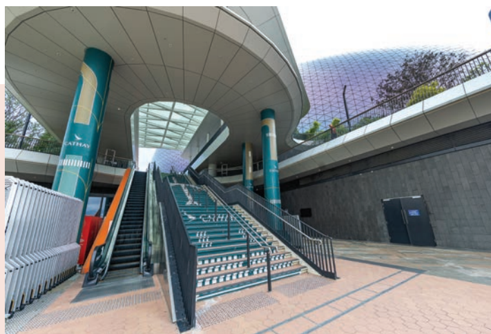
Kai Tak Sports Park – Lifts & Escalators Project
