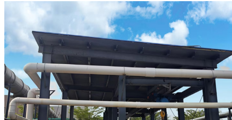
Wastewater Treatment Facility Upgrade
