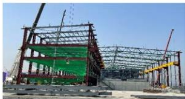
Figure 3: BPED and Electrical Control Room
