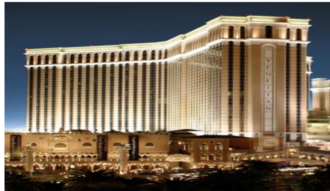
Figure 2: Venetian Hotel in Macau
