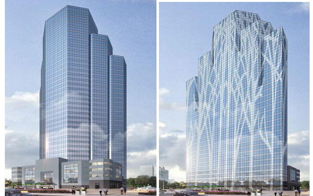
Figure 13: Proposed BIPV Renewal Project (LHS is Before Renewal and RHS is After Renewal)
