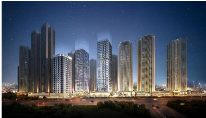
Figure 19: Coli's Residential Property Project One Blossom Cove in Guangzhou
