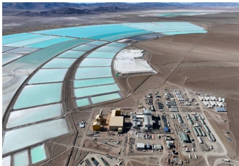
Figure 1: Olaroz Stage 2 - ponds fully commissioned
