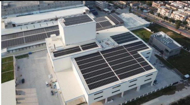
Figure 9: Unity's 600kW rooftop grid-connected solar PV project for Zhuhai Xiangbang's production plant
