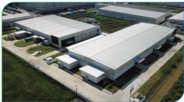
位於泰國春武里府安美德工業園的生產廠房。 Production facility located in Amata Industrial Estate, Chonburi, Thailand.
